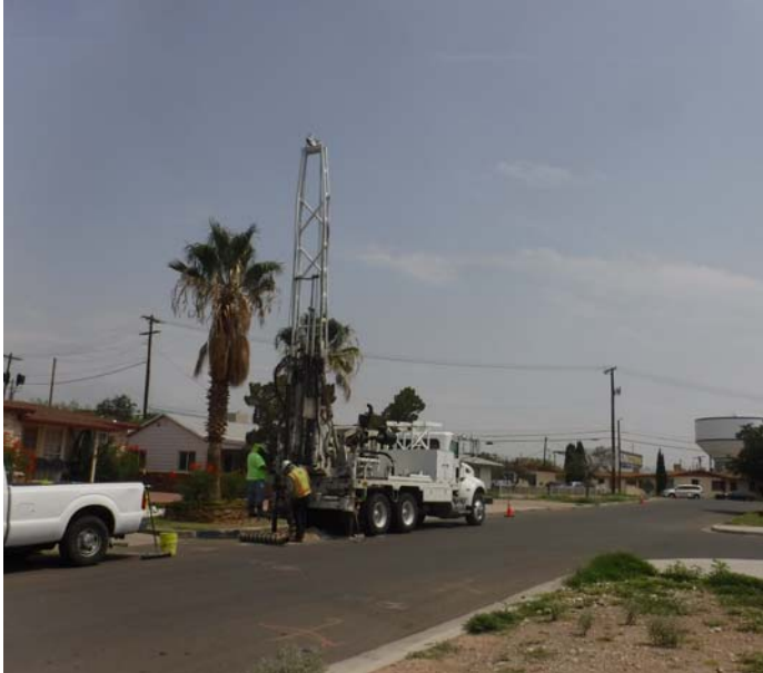
PHOTO NO. 25: General view of our subsurface soil drilling operations at vertical boring B-7.
