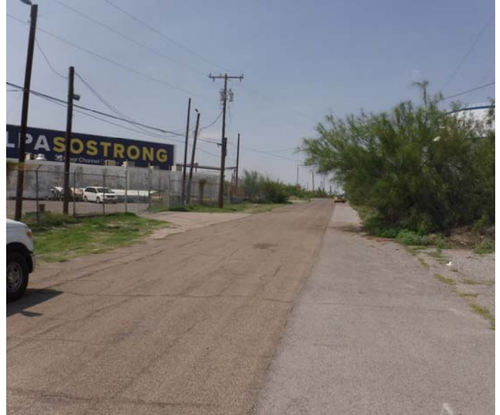
PHOTO NO. 18: General view of original pipeline route on Happer Street looking north.
