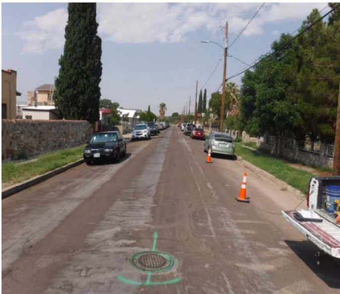
PHOTO NO. 3: General view of original pipeline route on Bishop Way looking southwest.
