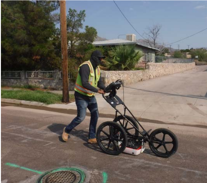
PHOTO NO. 33: General view of our ground penetrating radar operations on Bishop way.
