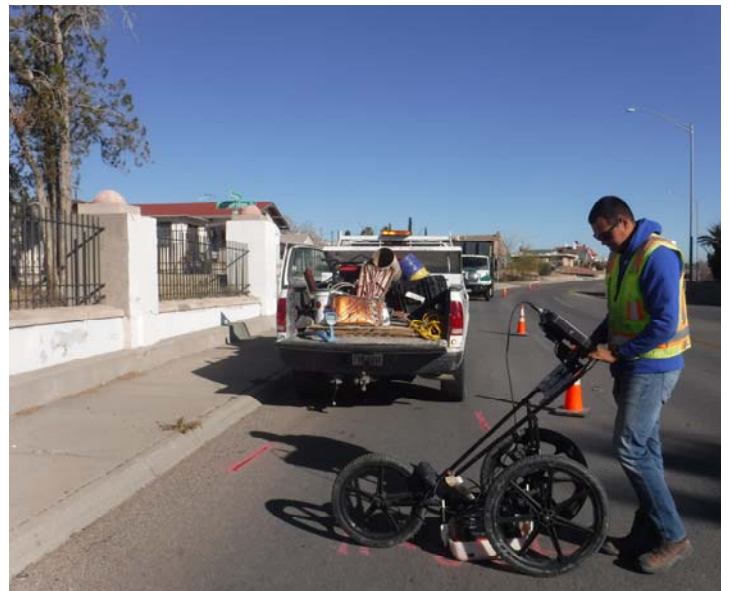
PHOTO NO. 40: General GPR utility locate activities at vertical boring B-11.
