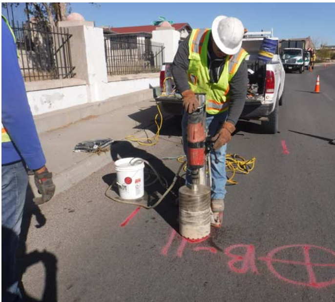
PHOTO NO. 43: General view of coring activities at vertical boring B-11.
