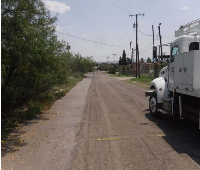
PHOTO NO. 19: General view of original pipeline route on Happer Street looking south.
