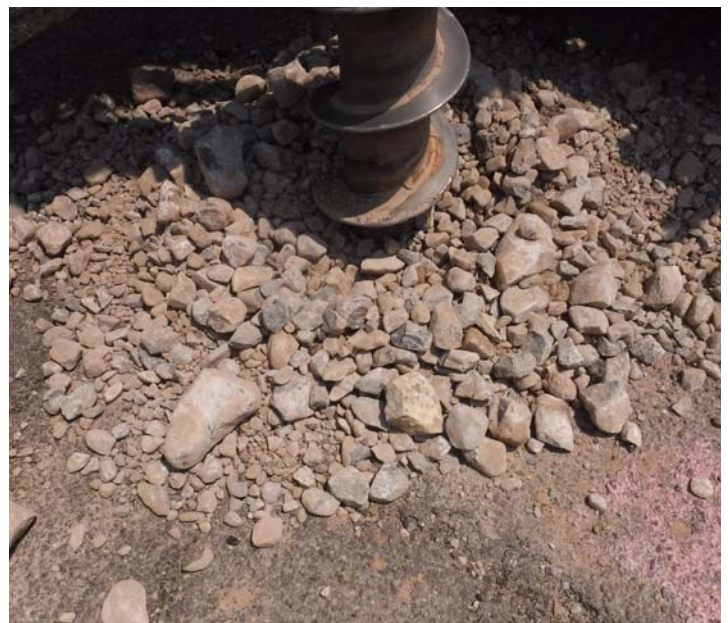
PHOTO NO. 32: General view of gravelly soils encountered in vertical boring B-10.
