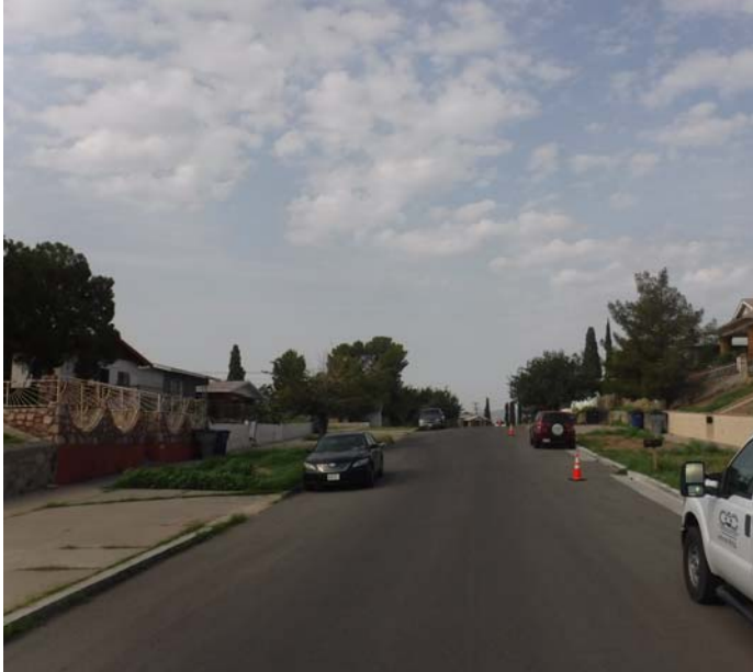
PHOTO NO. 7: General view of original pipeline route on Happer Street looking southwest.
