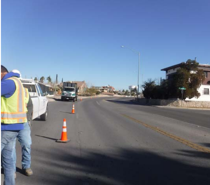
PHOTO NO. 37: General view of site existing pavement conditions at vertical boring location B-11 looking north.
