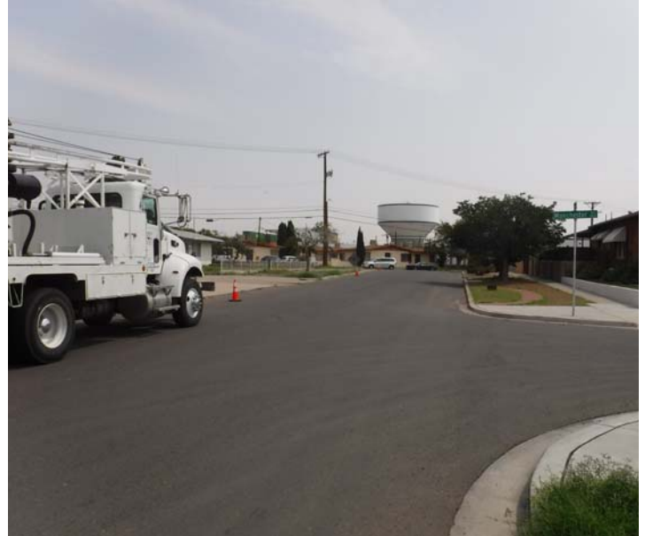
PHOTO NO. 14: General view of original pipeline route on Happer Street looking northeast.
