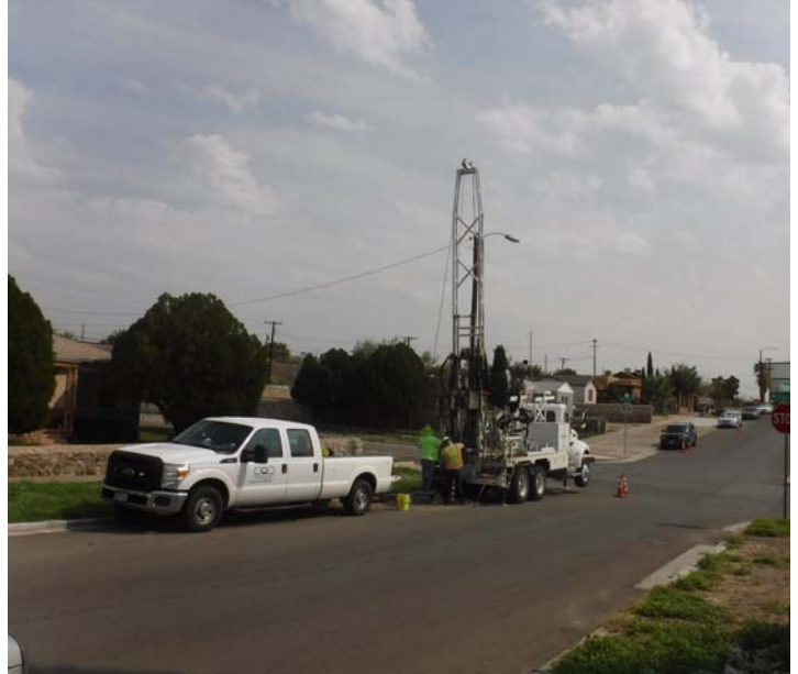
PHOTO NO. 24: General view of our subsurface soil drilling operations at vertical boring B-6.
