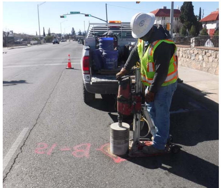
PHOTO NO. 44: General view of coring activities at vertical boring B-12.
