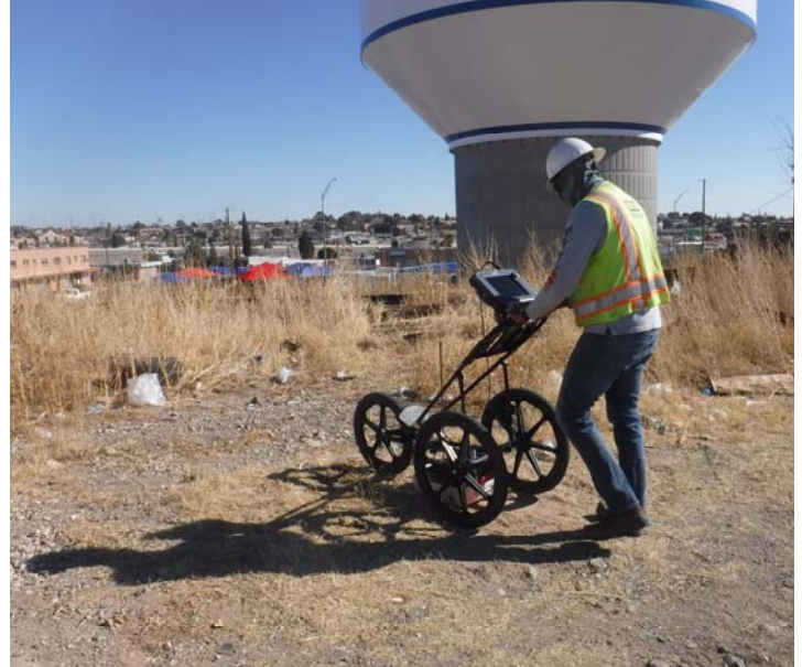
PHOTO NO. 42: General GPR utility locate activities at vertical boring B-13.
