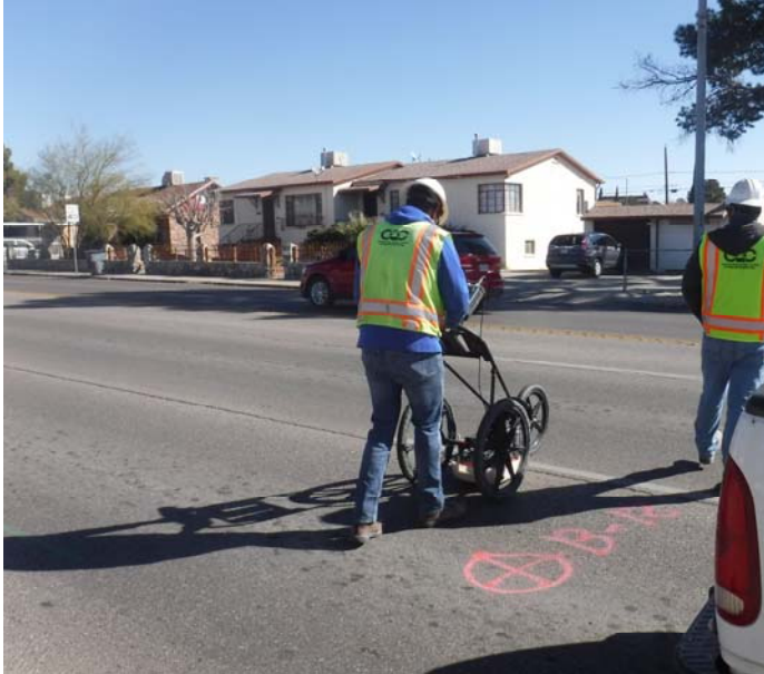
PHOTO NO. 41: General GPR utility locate activities at vertical boring B-12.
